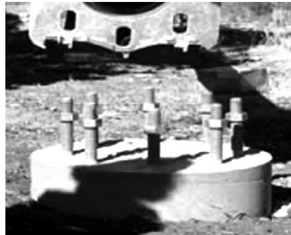
A typical pier foundation
